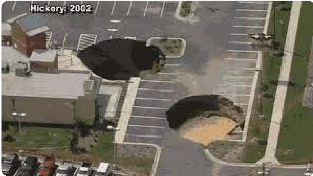
History and Repair of Buffalo's Sinkhole in Hickory, NC
