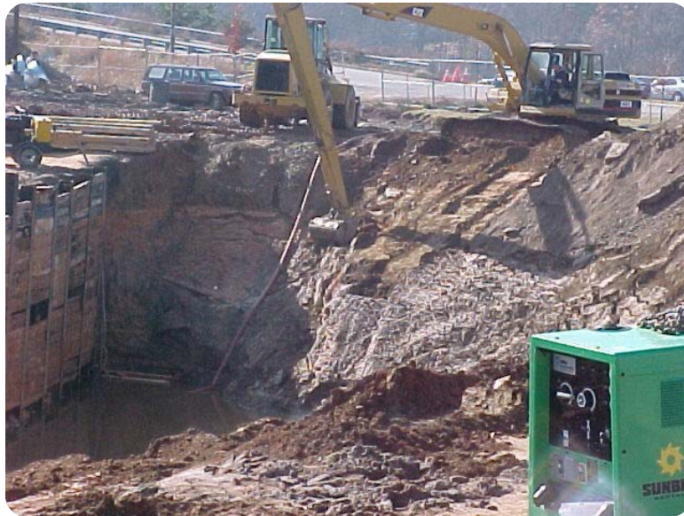
History and Repair of Buffalo's Sinkhole in Hickory, NC
