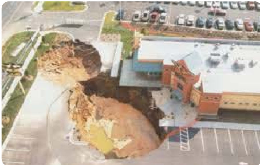
History and Repair of Buffalo's Sinkhole in Hickory, NC
